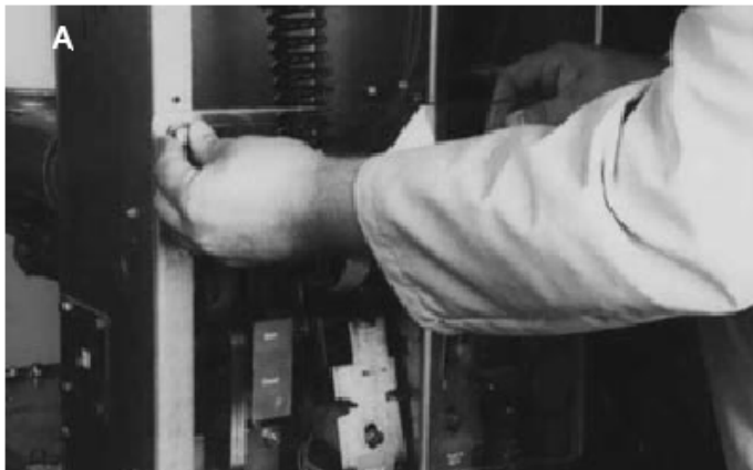
Figure 6-9 Attaching CloSure™ Test Tool at Hole "A"
